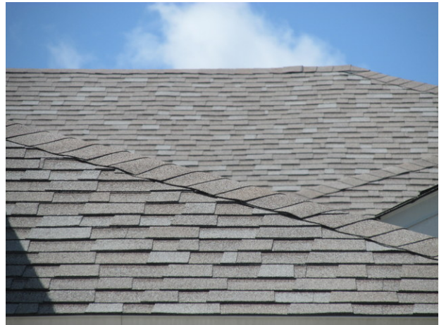
Asphalt shingle roof at villa unit
