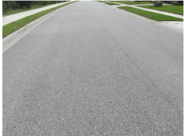
Typical good condition of asphalt pavement
