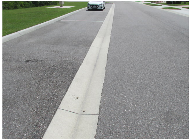
Typical condition of concrete gutters
