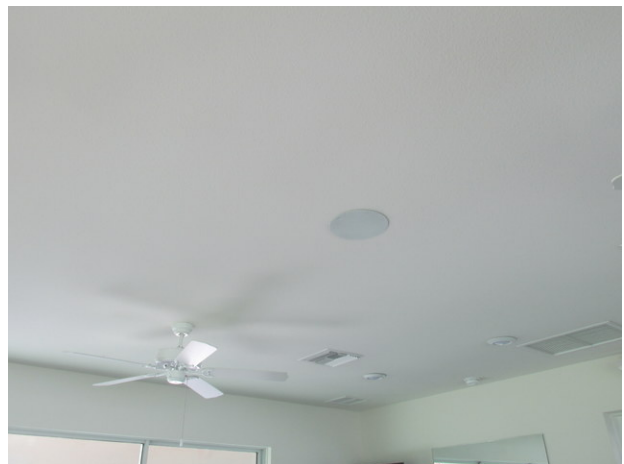
Finishes and ceiling fan at exercise room
