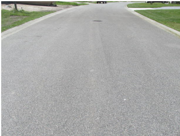
Typical good condition of asphalt pavement
