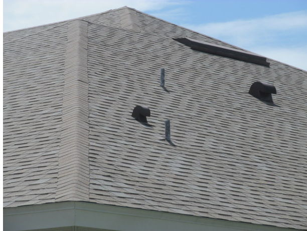
Asphalt shingle roof at villa unit
