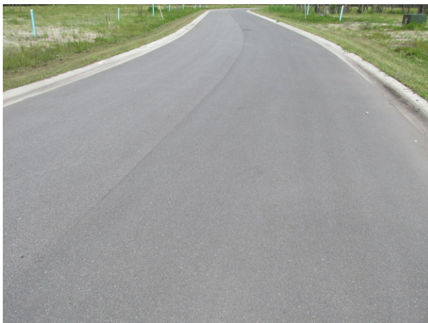
Typical good condition of asphalt pavement
