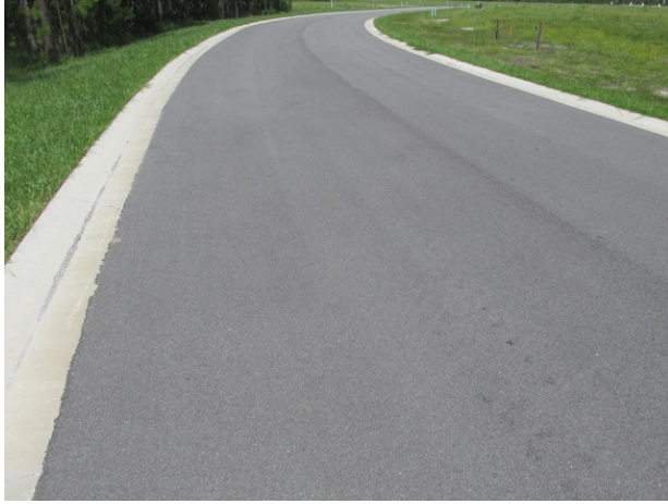
Typical good condition of asphalt pavement
