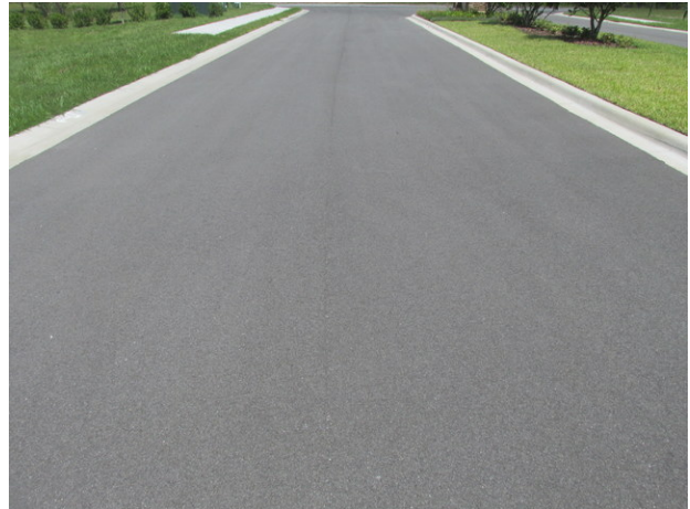
Typical good condition of asphalt pavement
