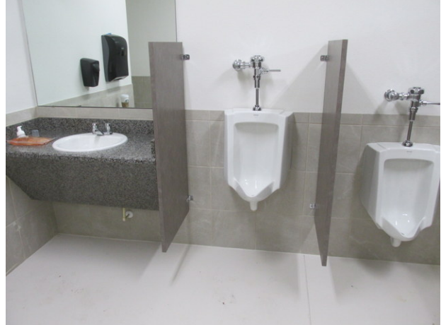
Finishes and fixtures at rest room
