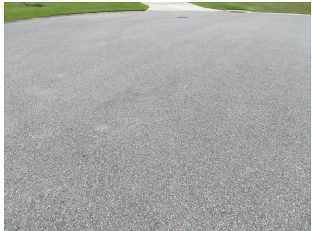
Typical good condition of asphalt pavement
