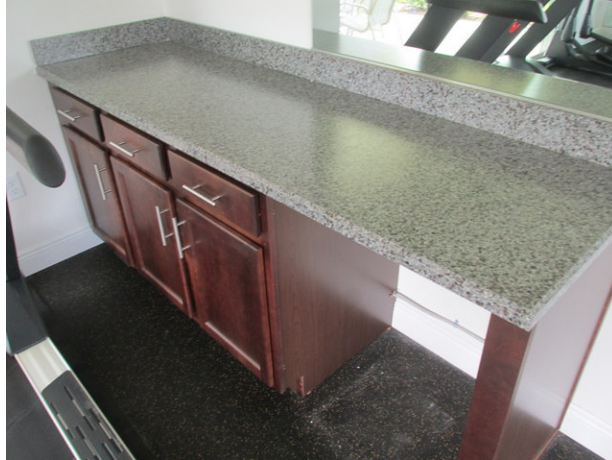
Cabinets and countertop at exercise room
