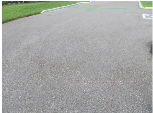
Asphalt pavement at clubhouse parking area
