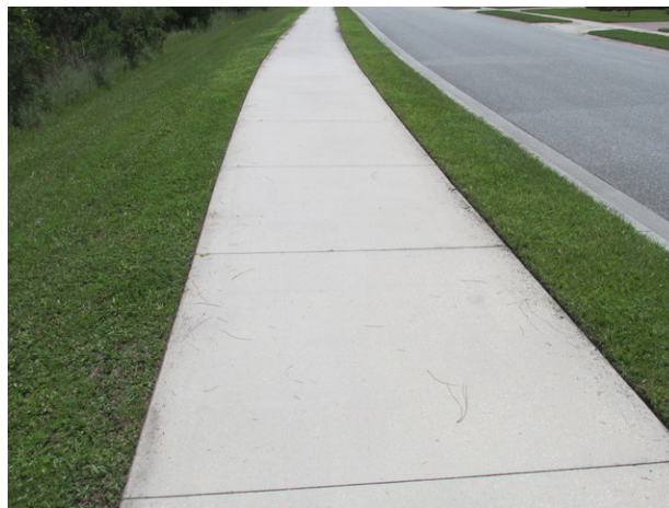
Typical condition of concrete sidewalks
