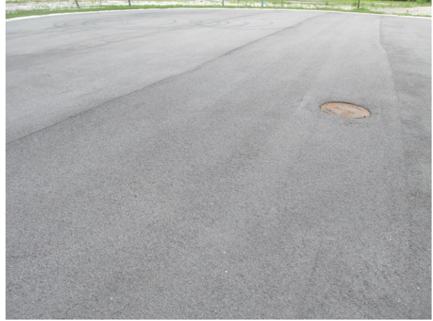
Typical good condition of asphalt pavement
