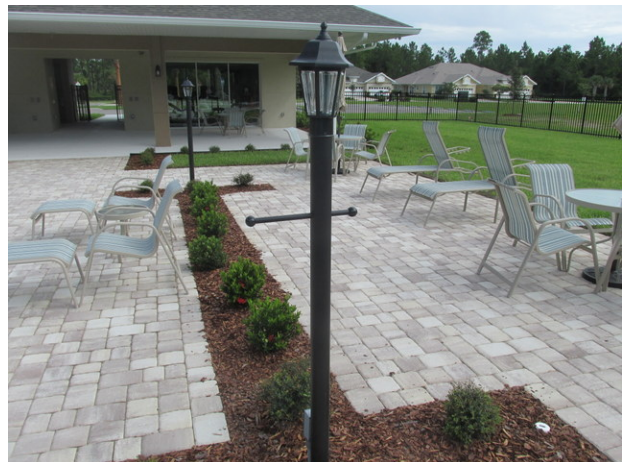
Light poles and fixtures at pool area
