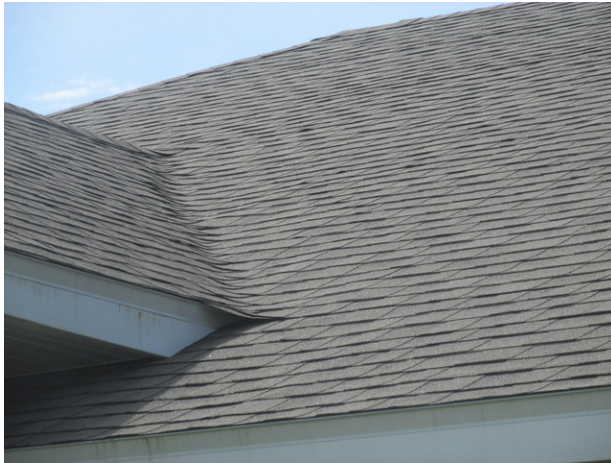
Asphalt shingle roof at clubhouse
