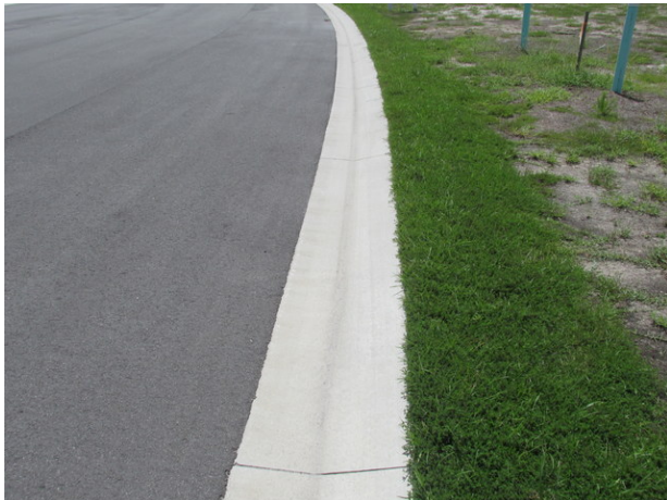
Typical condition of concrete gutters
