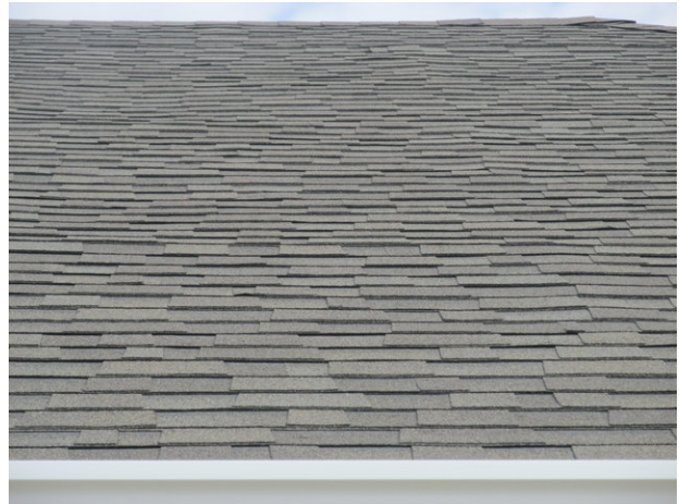
Asphalt shingle roof at clubhouse
