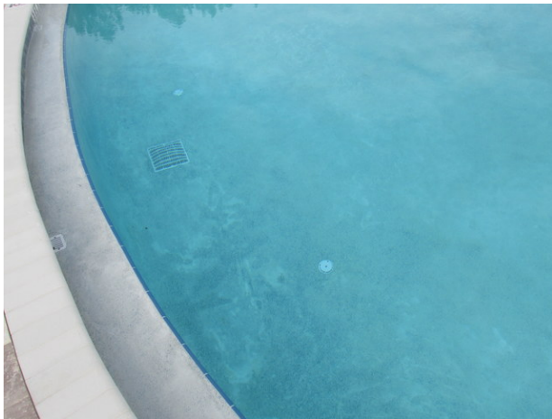
Pool plaster finish
