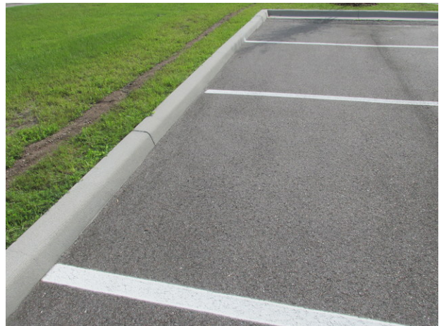
Concrete curb at clubhouse parking area
