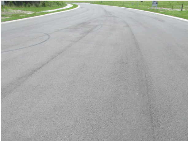
Typical good condition of asphalt pavement
