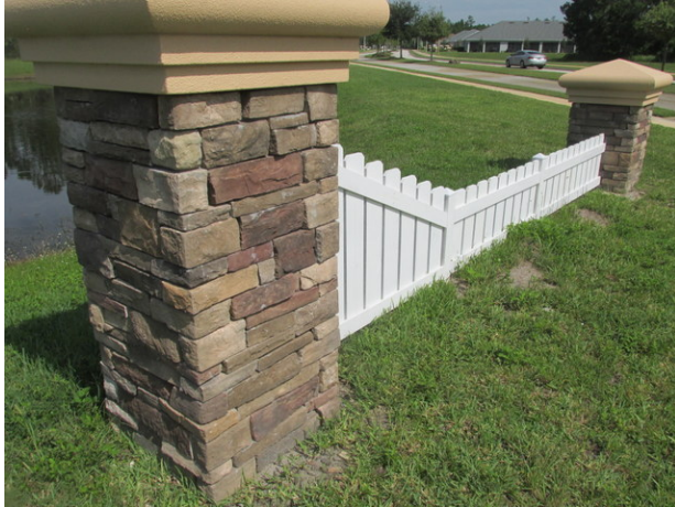
Stone veneer columns and wood fence
