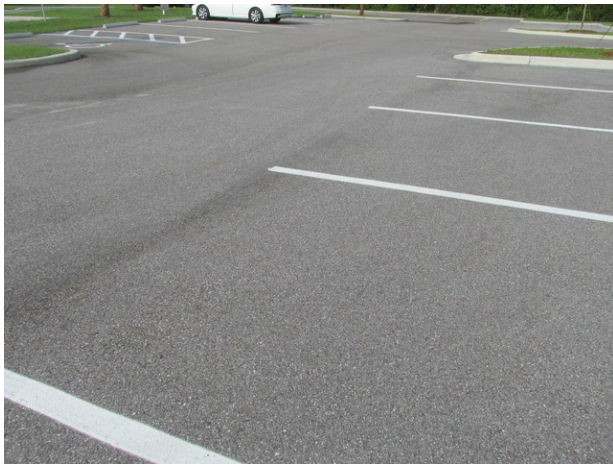
Asphalt pavement at clubhouse parking area
