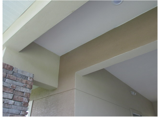
Finishes at clubhouse exterior
