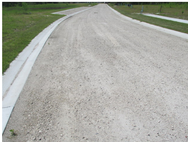
Asphalt pavement street under construction
