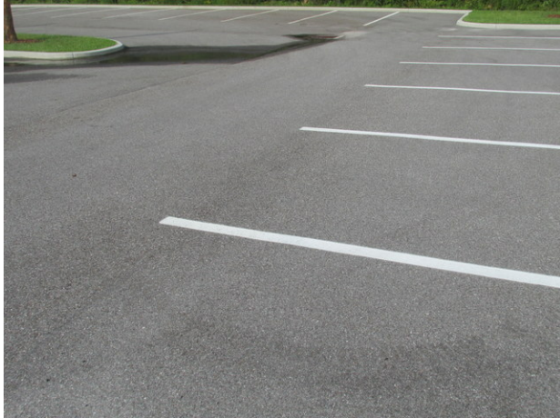
Asphalt pavement at clubhouse parking area
