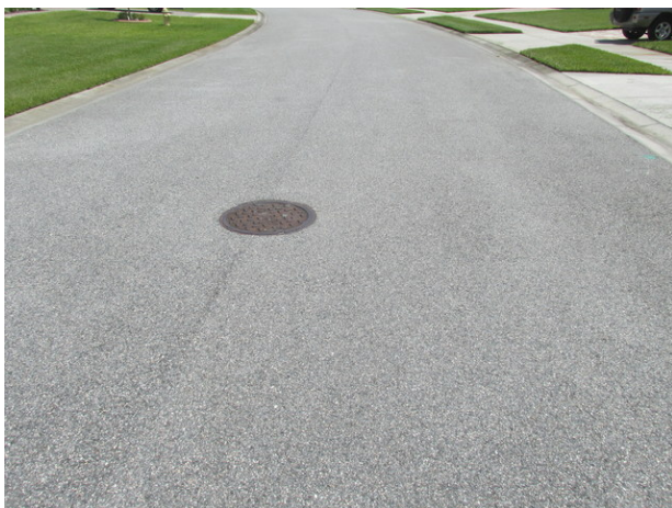
Typical good condition of asphalt pavement
