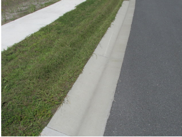
Typical condition of concrete gutters
