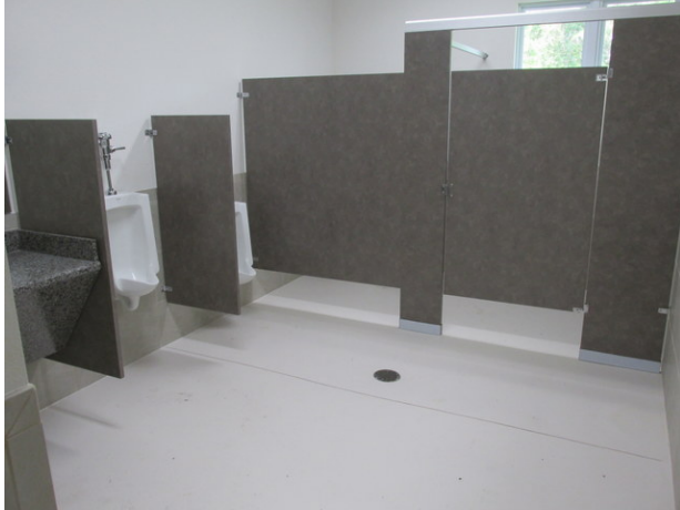
Finishes and fixtures at rest room
