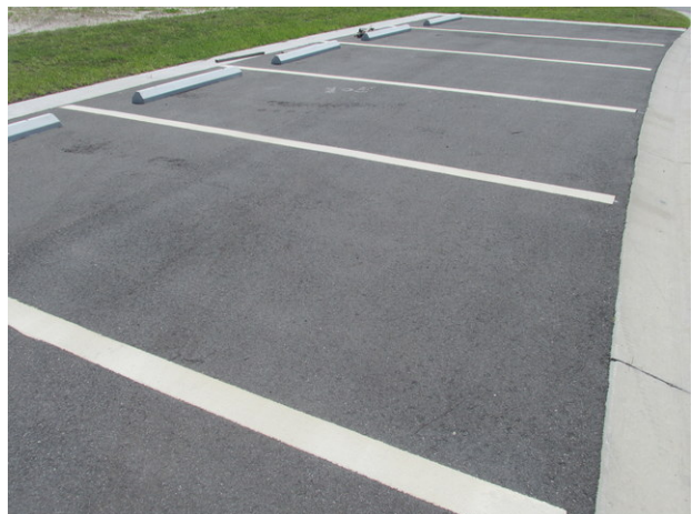
Typical good condition of asphalt pavement
