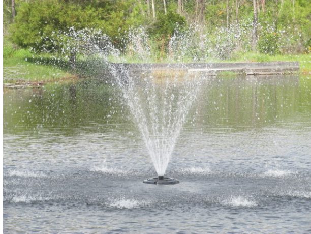
Aerator at pond
