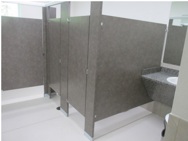
Finishes and fixtures at rest room
