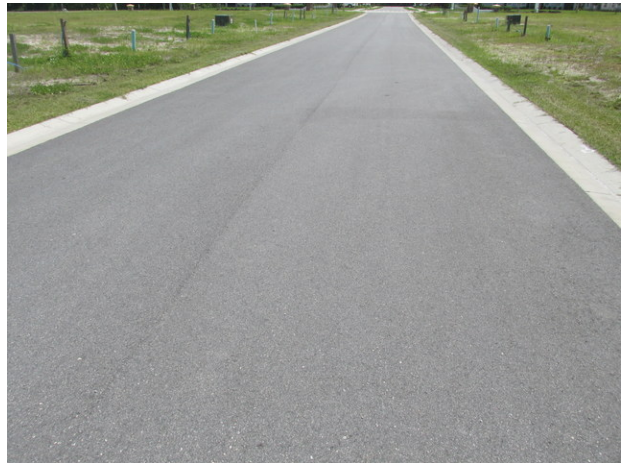
Typical good condition of asphalt pavement
