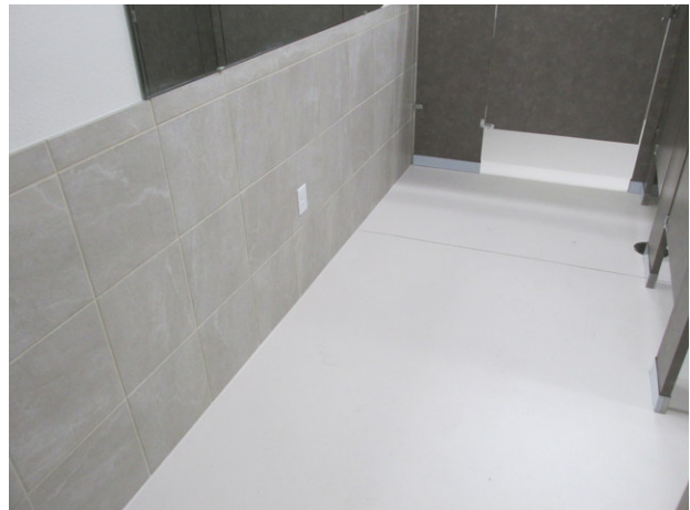
Tile wall coverings and coated floor at rest room
