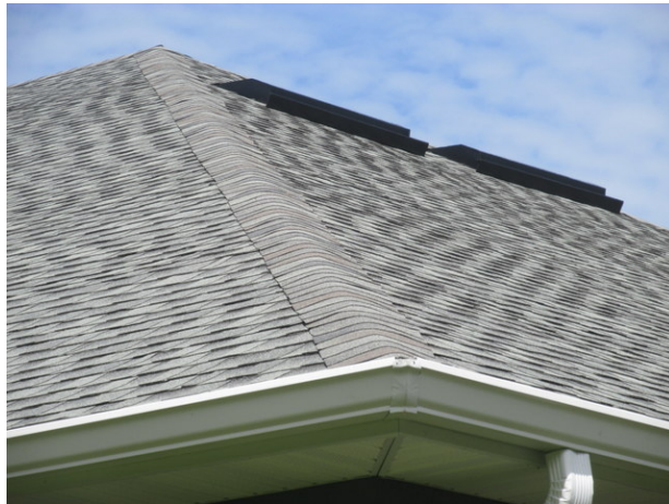
Asphalt shingle roof at villa unit
