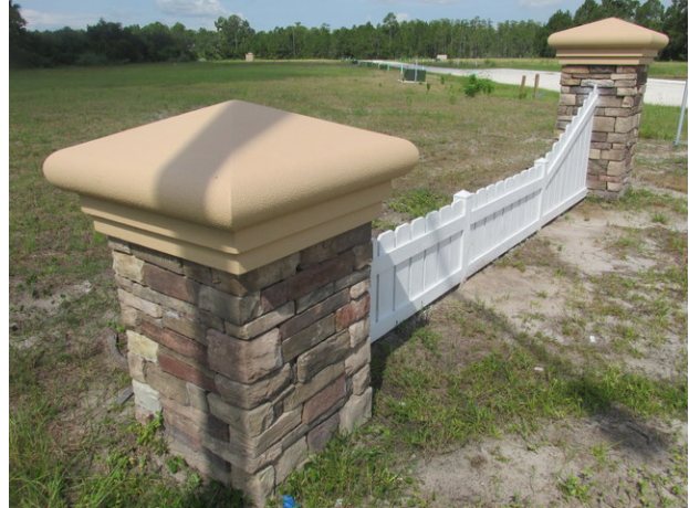
Stone veneer columns and wood fence
