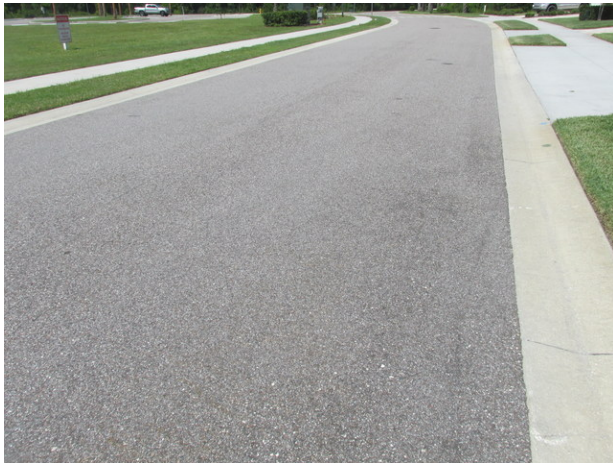
Typical good condition of asphalt pavement
