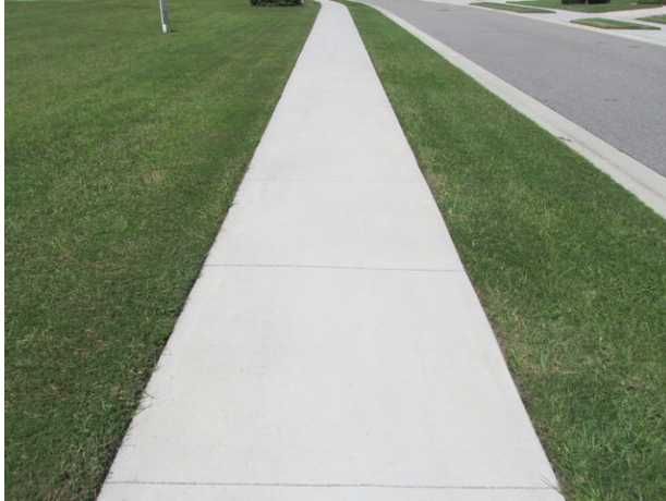
Typical condition of concrete sidewalks
