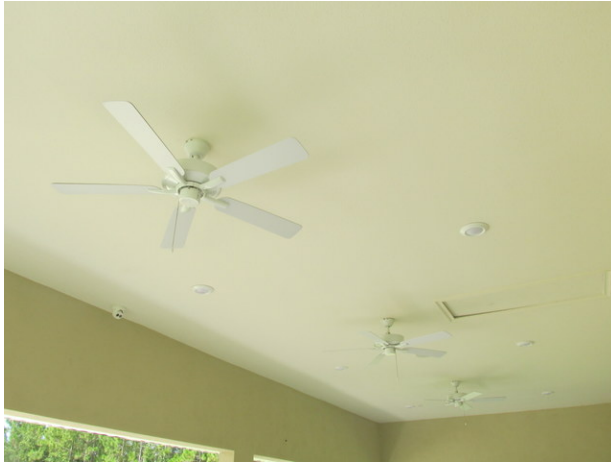
Finishes at clubhouse exterior
