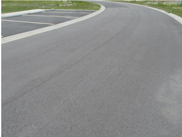
Typical good condition of asphalt pavement
