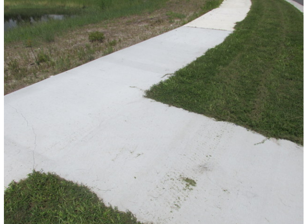
Typical condition of concrete sidewalks
