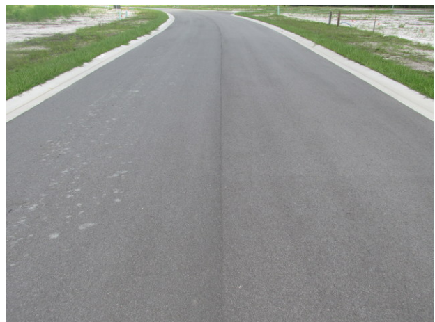
Typical good condition of asphalt pavement
