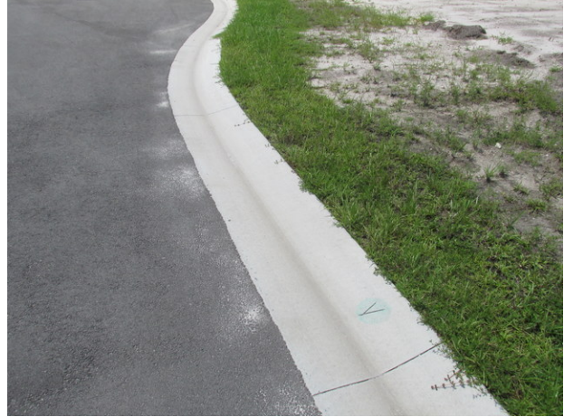
Typical condition of concrete gutters
