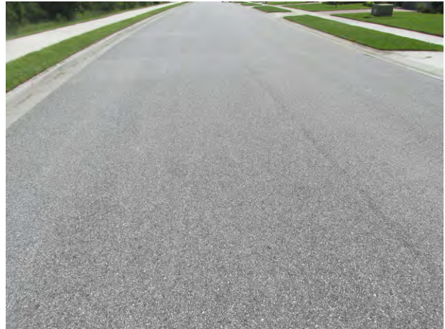
Typical good condition of asphalt pavement
