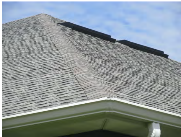
Asphalt shingle roof at villa unit
