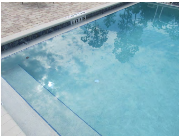
Pool plaster finish, waterline tile and accent tile
