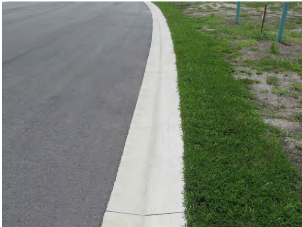
Typical condition of concrete gutters
