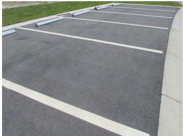
Typical good condition of asphalt pavement
