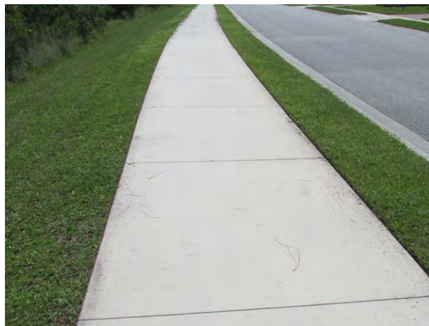
Typical condition of concrete sidewalks
