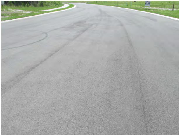
Typical good condition of asphalt pavement
