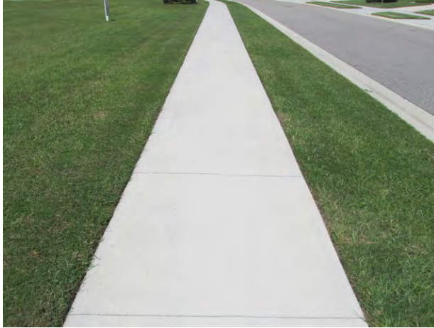
Typical condition of concrete sidewalks
