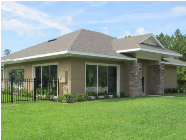
Exterior view of clubhouse
