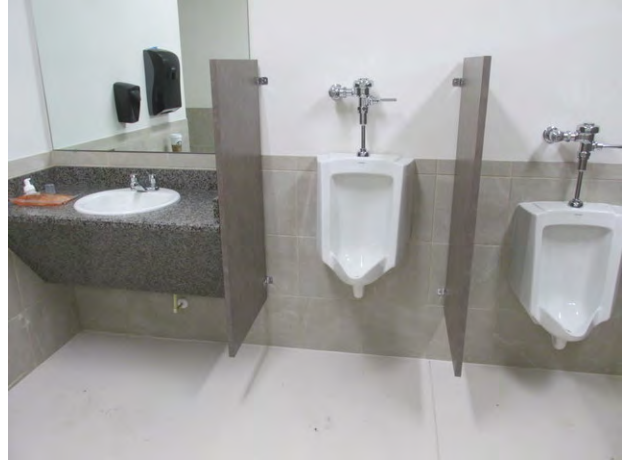
Finishes and fixtures at rest room
