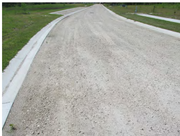
Asphalt pavement street under construction
