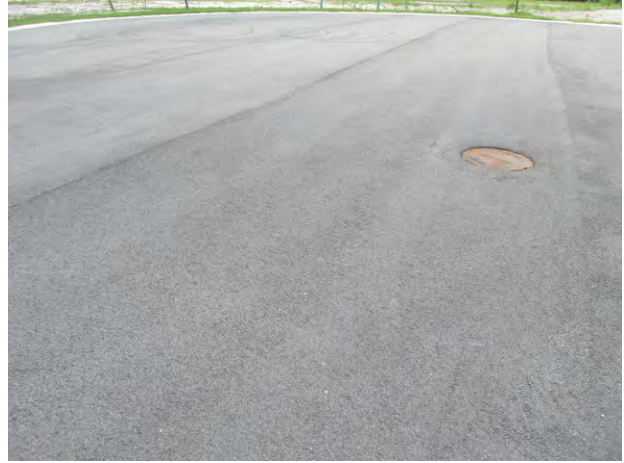
Typical good condition of asphalt pavement
