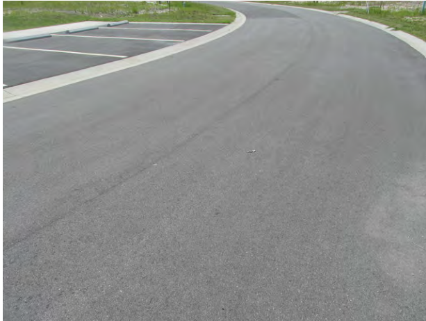
Typical good condition of asphalt pavement
