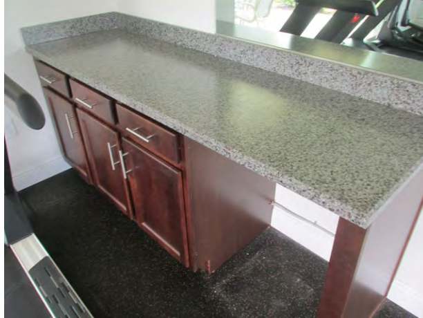
Cabinets and countertop at exercise room
