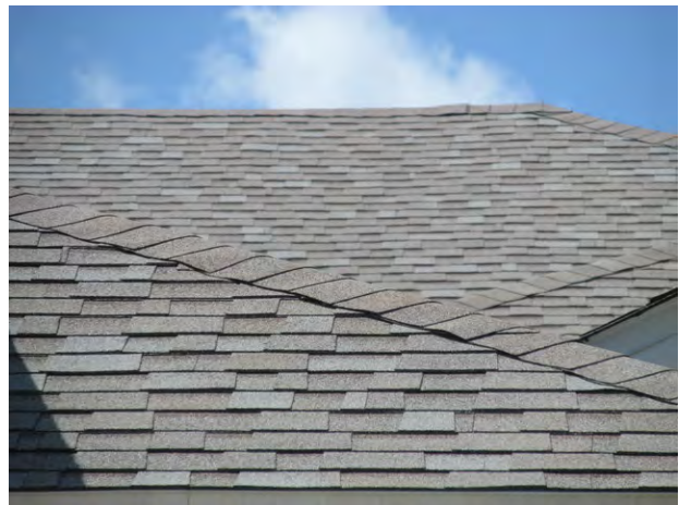
Asphalt shingle roof at villa unit
