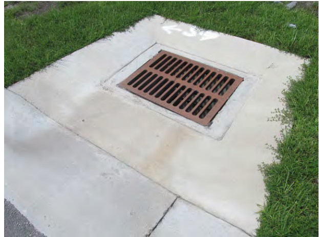
Catch basin and concrete collar
