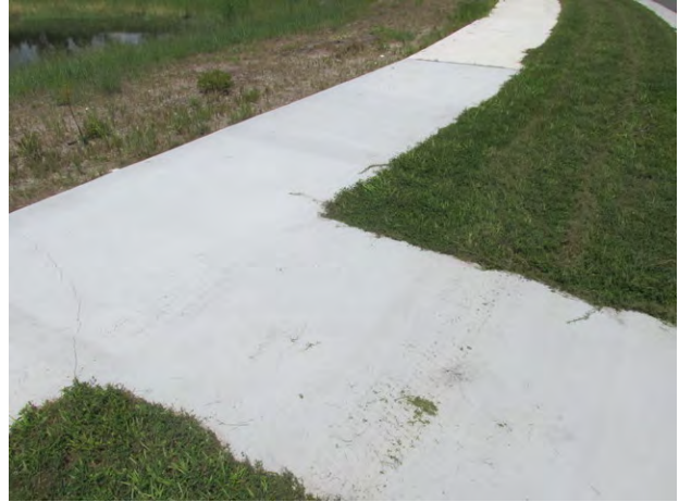
Typical condition of concrete sidewalks
