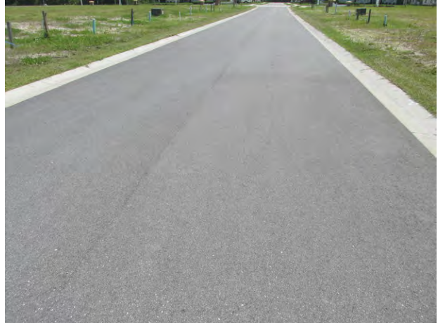
Typical good condition of asphalt pavement
