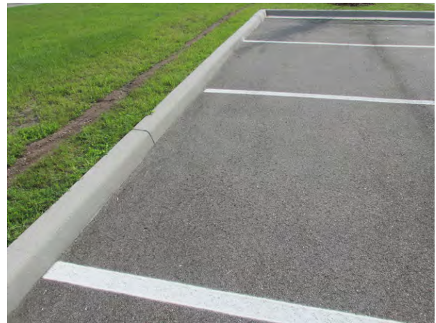
Concrete curb at clubhouse parking area
