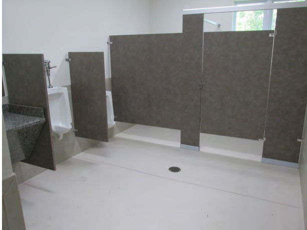
Finishes and fixtures at rest room
