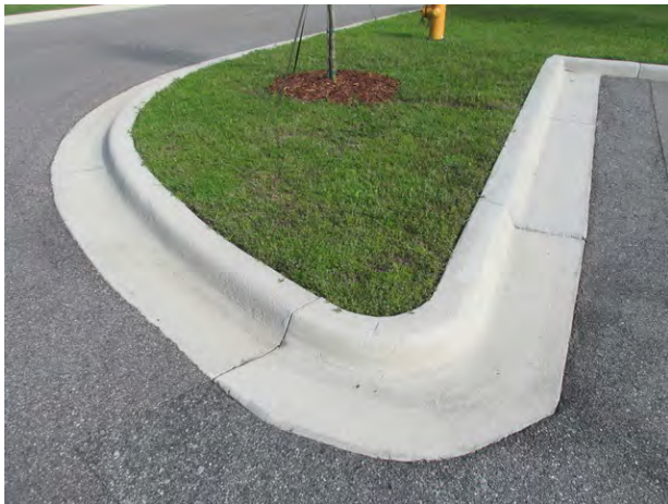
Concrete curb and gutter at clubhouse parking area
