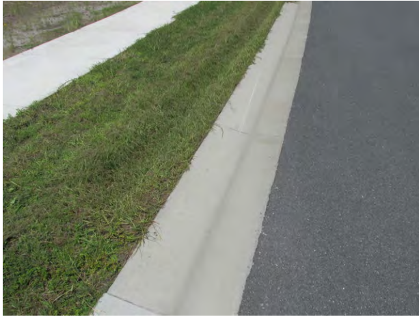
Typical condition of concrete gutters
