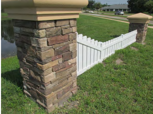
Stone veneer columns and wood fence
