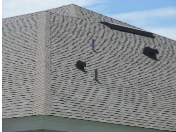
Asphalt shingle roof at villa unit
