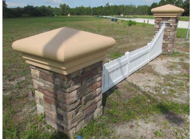
Stone veneer columns and wood fence
