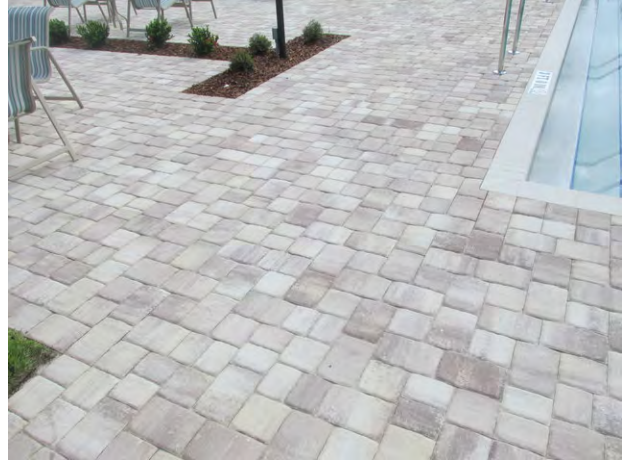
Pavers at pool deck
