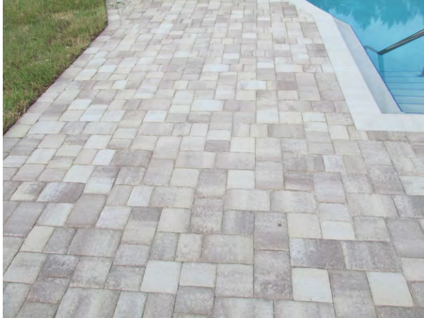
Pavers at pool deck
