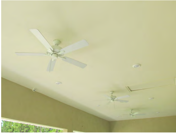
Finishes at clubhouse exterior
