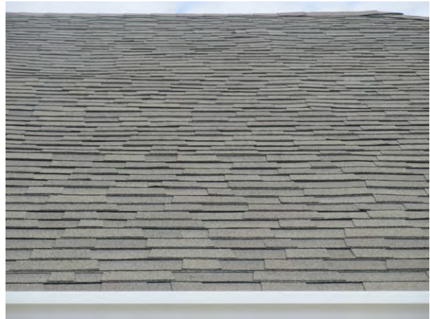
Asphalt shingle roof at clubhouse
