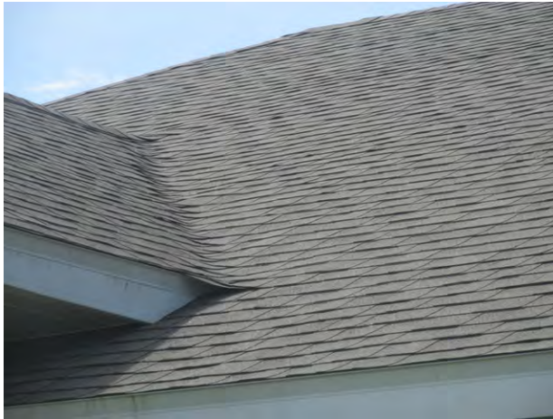
Asphalt shingle roof at clubhouse
