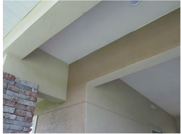
Finishes at clubhouse exterior
