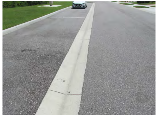
Typical condition of concrete gutters
