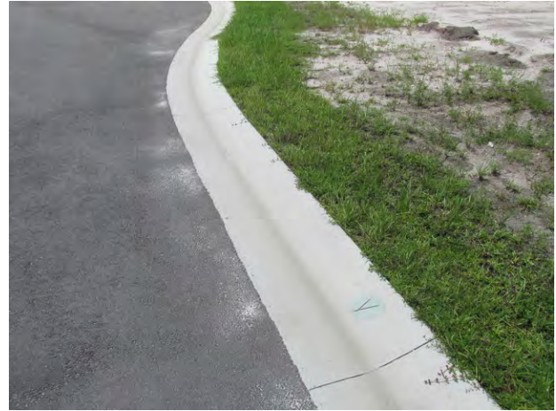
Typical condition of concrete gutters
