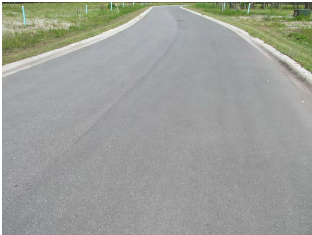
Typical good condition of asphalt pavement
