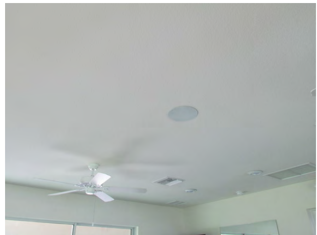
Finishes and ceiling fan at exercise room
