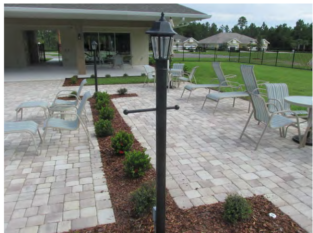
Light poles and fixtures at pool area
