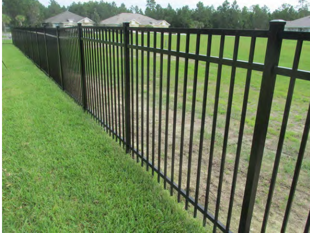
Aluminum fence at pool area
