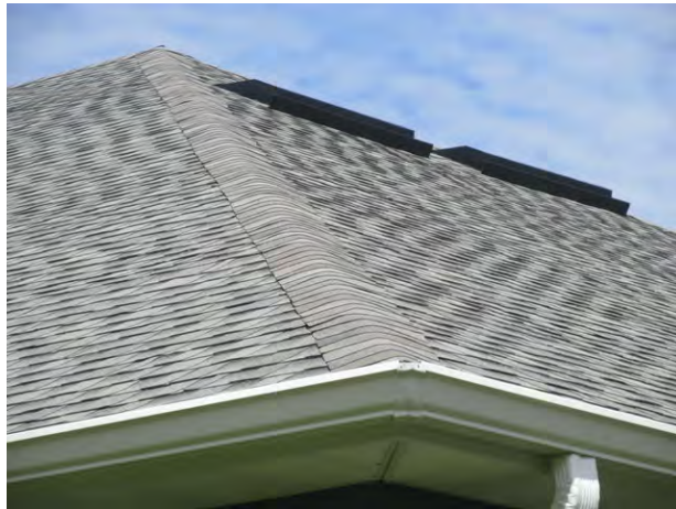
Asphalt shingle roof at villa unit
