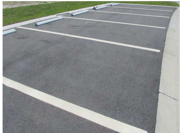
Typical good condition of asphalt pavement
