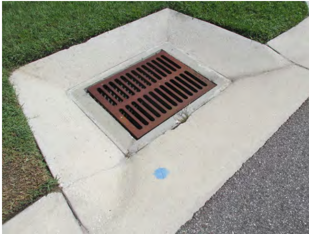
Catch basin and concrete collar
