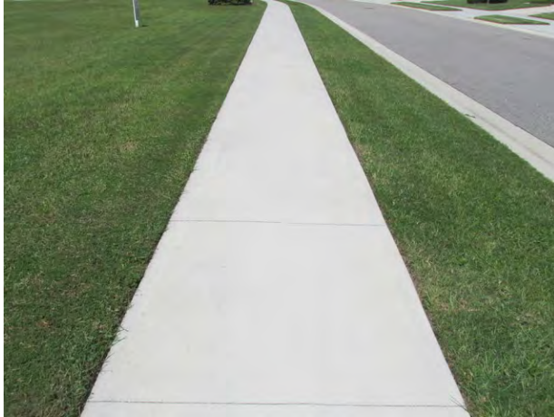
Typical condition of concrete sidewalks
