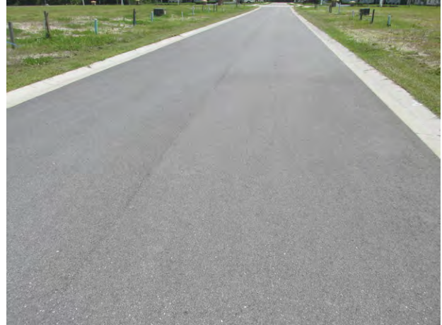
Typical good condition of asphalt pavement
