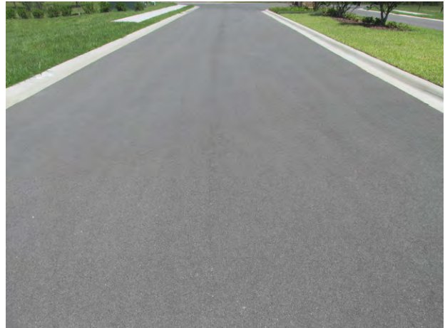
Typical good condition of asphalt pavement
