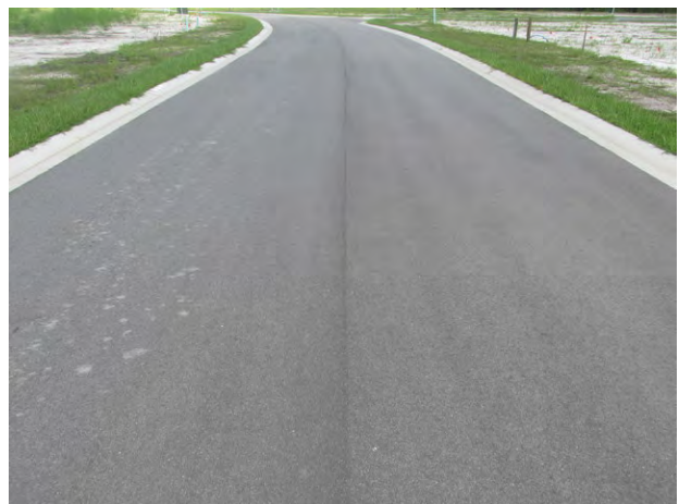
Typical good condition of asphalt pavement
