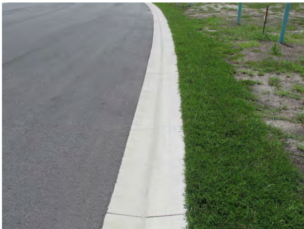
Typical condition of concrete gutters
