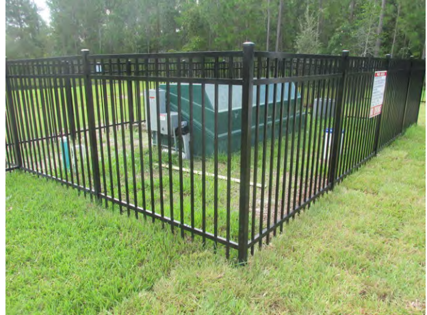
Aluminum fence at pool area
