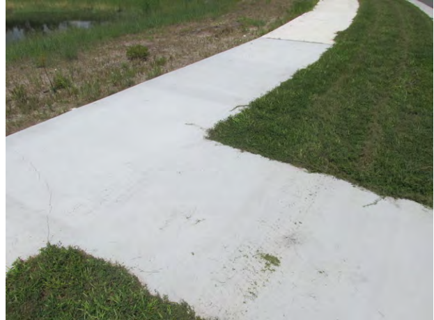
Typical condition of concrete sidewalks
