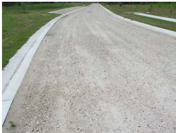
Asphalt pavement street under construction
