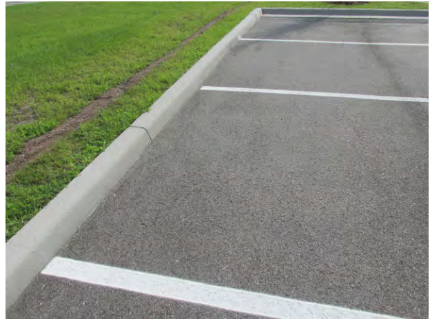
Concrete curb at clubhouse parking area
