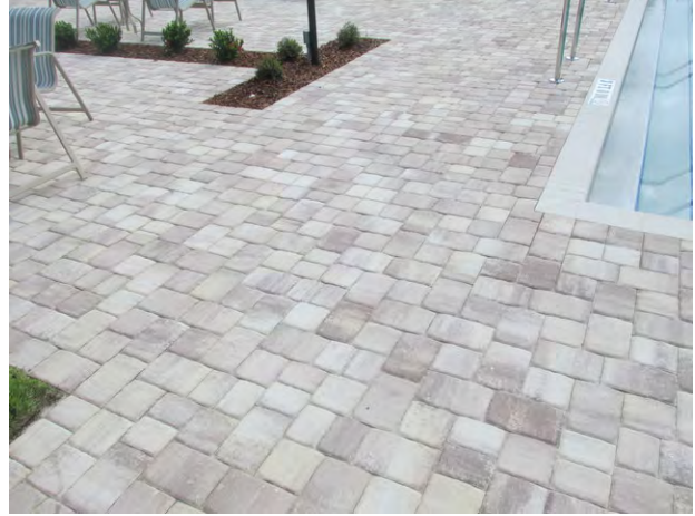
Pavers at pool deck
