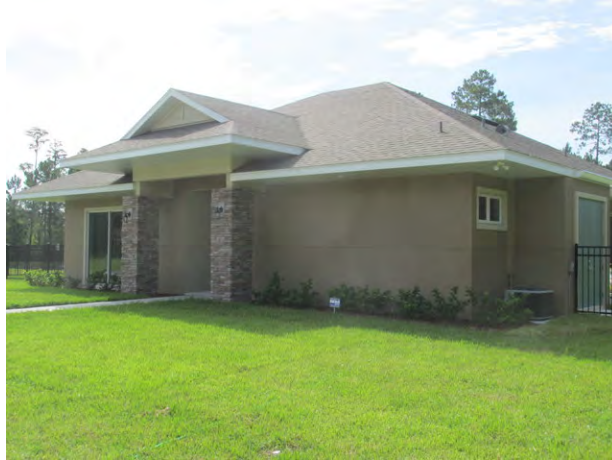
Exterior view of clubhouse
