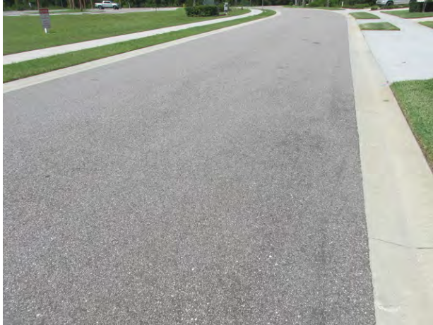
Typical good condition of asphalt pavement
