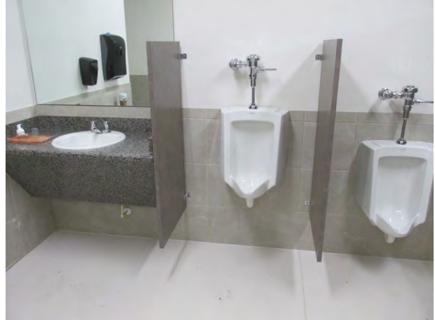
Finishes and fixtures at rest room
