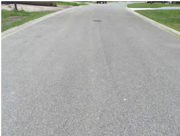
Typical good condition of asphalt pavement
