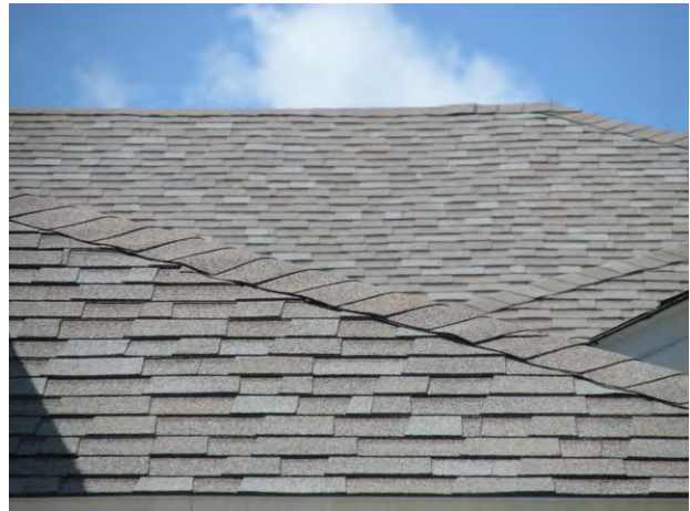
Asphalt shingle roof at villa unit
