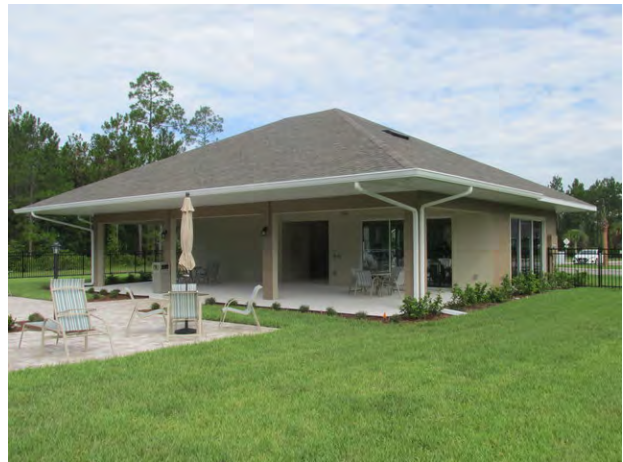
Exterior view of clubhouse
