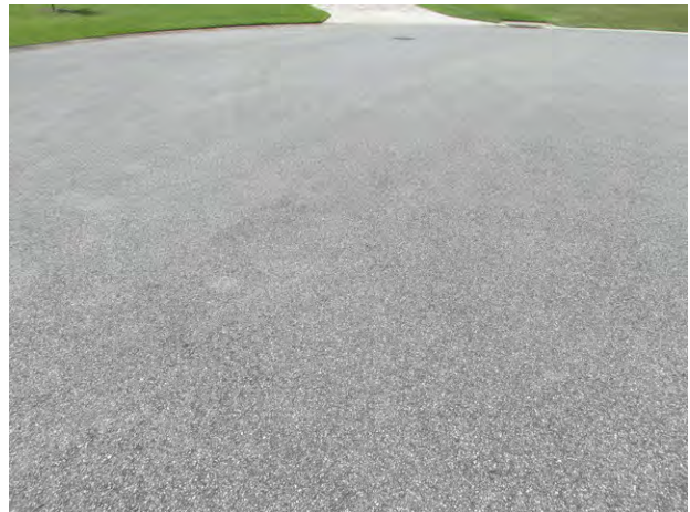
Typical good condition of asphalt pavement
