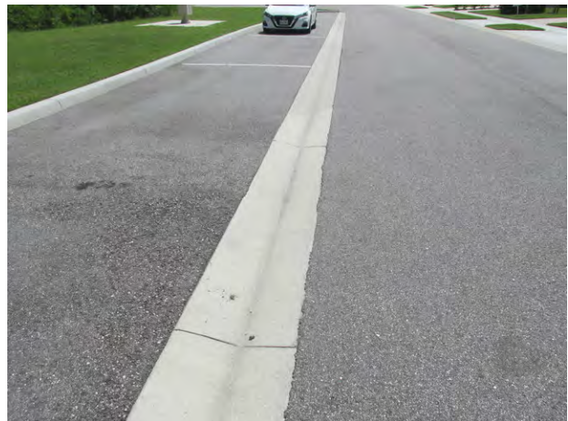
Typical condition of concrete gutters
