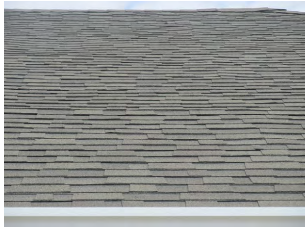
Asphalt shingle roof at clubhouse
