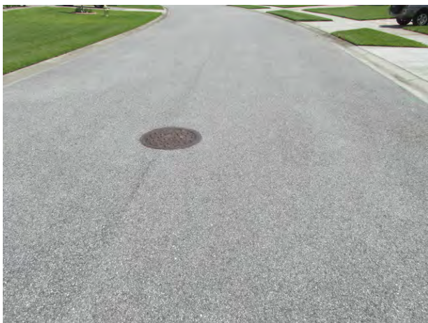
Typical good condition of asphalt pavement
