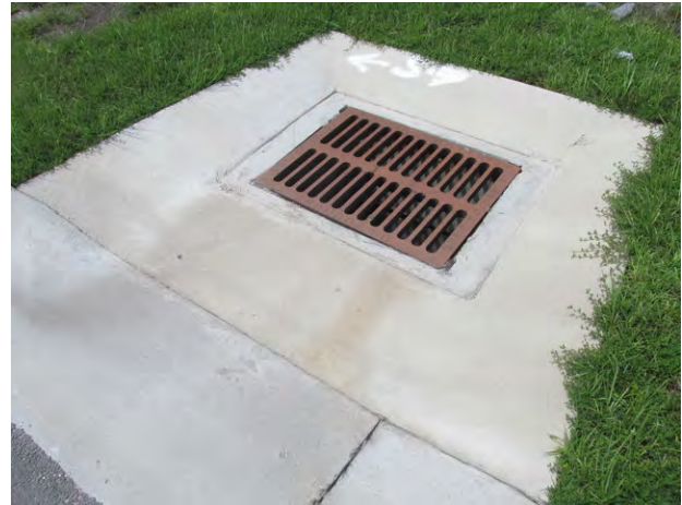
Catch basin and concrete collar
