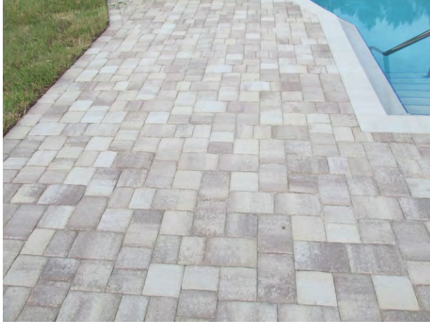
Pavers at pool deck
