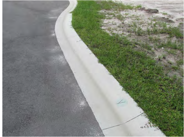
Typical condition of concrete gutters
