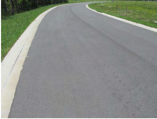
Typical good condition of asphalt pavement
