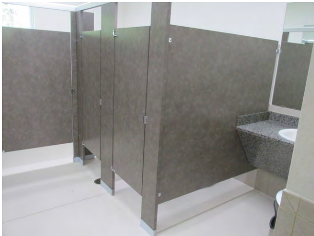
Finishes and fixtures at rest room
